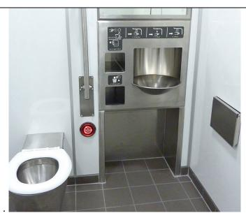
Toilet pans are wall-mounted to aid cleaning of the floors and removing silicone that can harbour germs and dirt and are manufactured out of stainless steel for strength and ease of cleaning.
